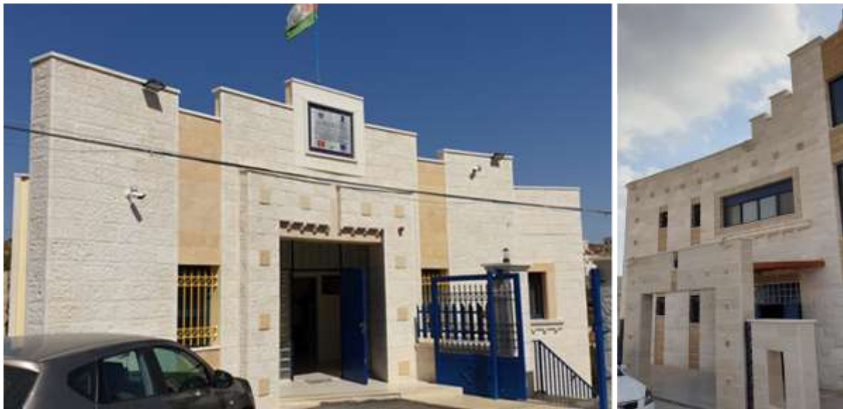
Figure 2 External façade of Marah Ma'allah (left) and Daher Al 'Abed (right) buildings
