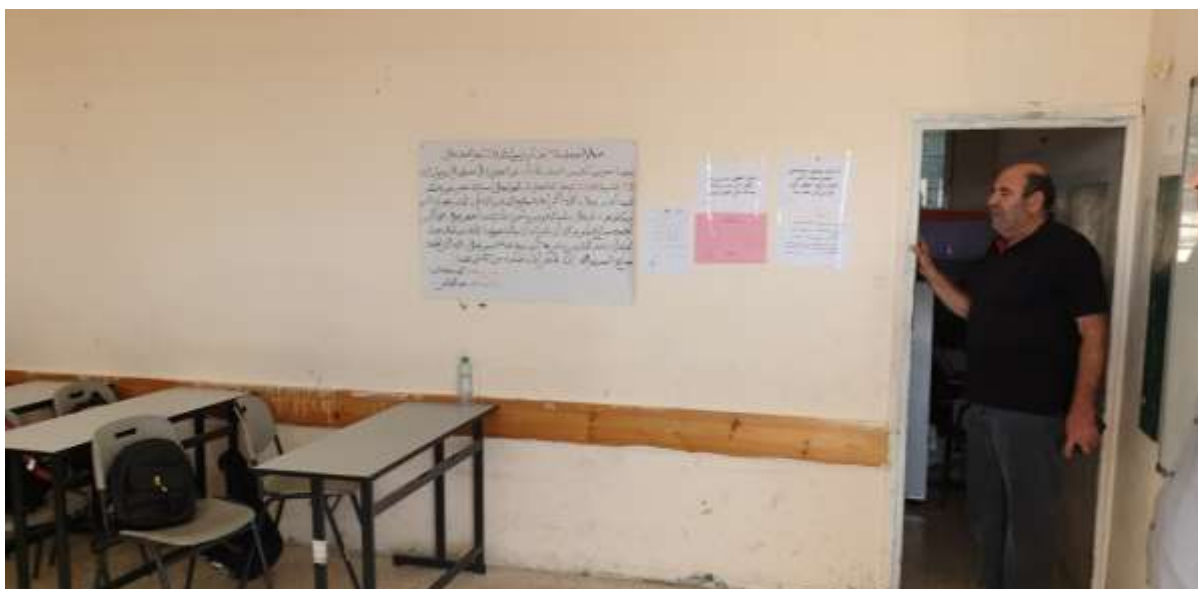
Figure 5 The dual classroom in Al Manshiya school before the extension
