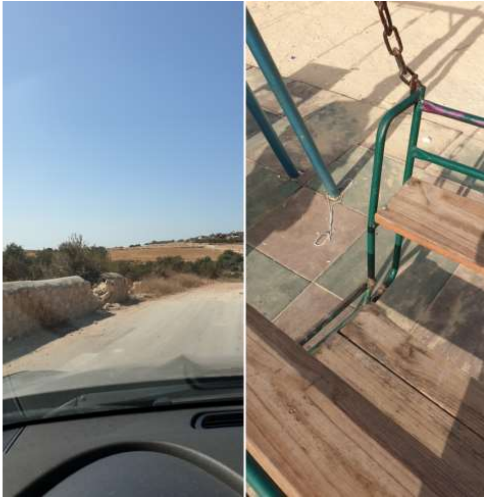
Figure 7 Deficiencies in Idna North Road and Daher Al 'Abed Park
