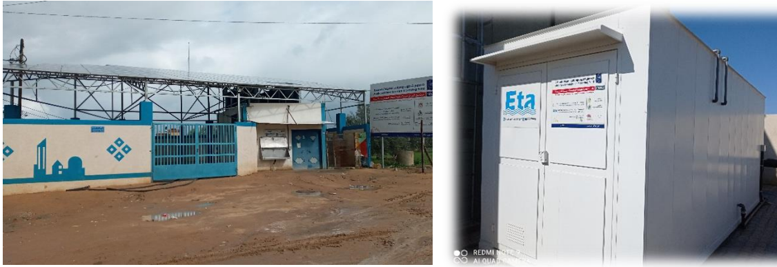
Figure 13: Establishing municipal brackish water RO desalination plants with PV System
