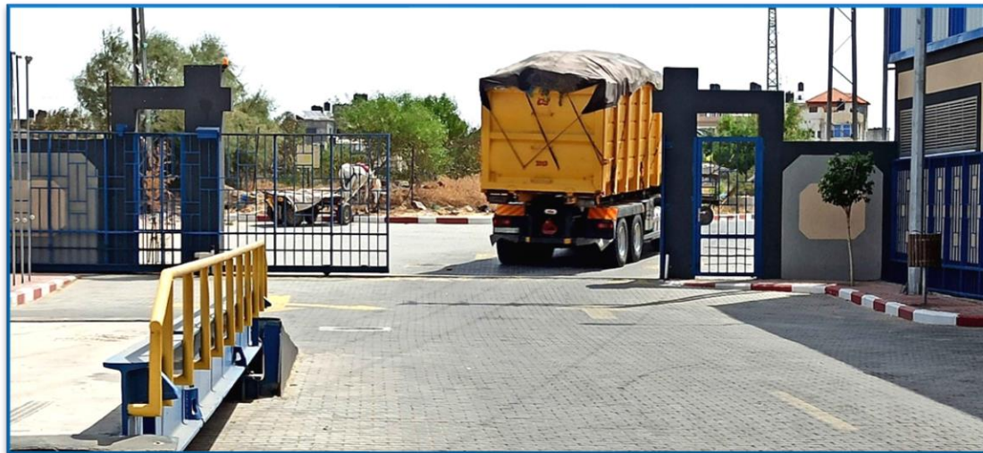
Top: drone photo of Rafah Transfer Station Compound (December 2019) Middle: animal collection cart coming into the transfer station (June 2020) Bottom: solid waste transfer truck leaving the transfer station (June 2020)
