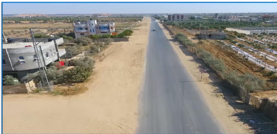
Access Road of Al-Fukhary (Sofa) Landfill
