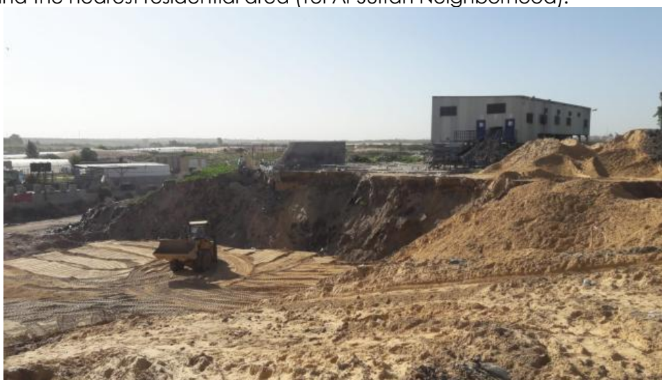
Construction of Rafah transfer station (December 2018)
