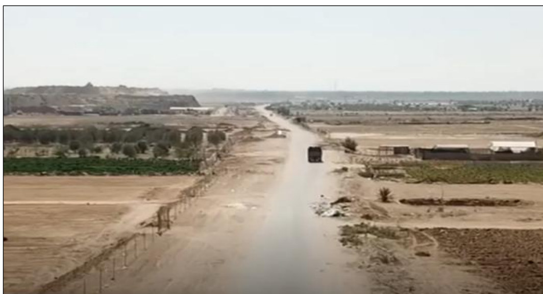
Al-Fukhary Landfill Access Road before the rehabilitation works (September 2018)
