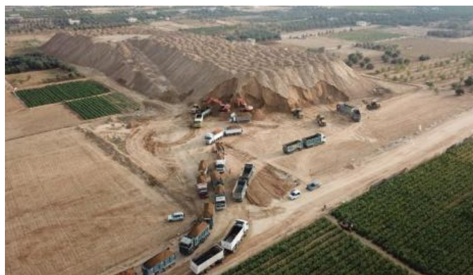
Removal and transfer of excavated material from the temporary stockpile to the final disposal site
