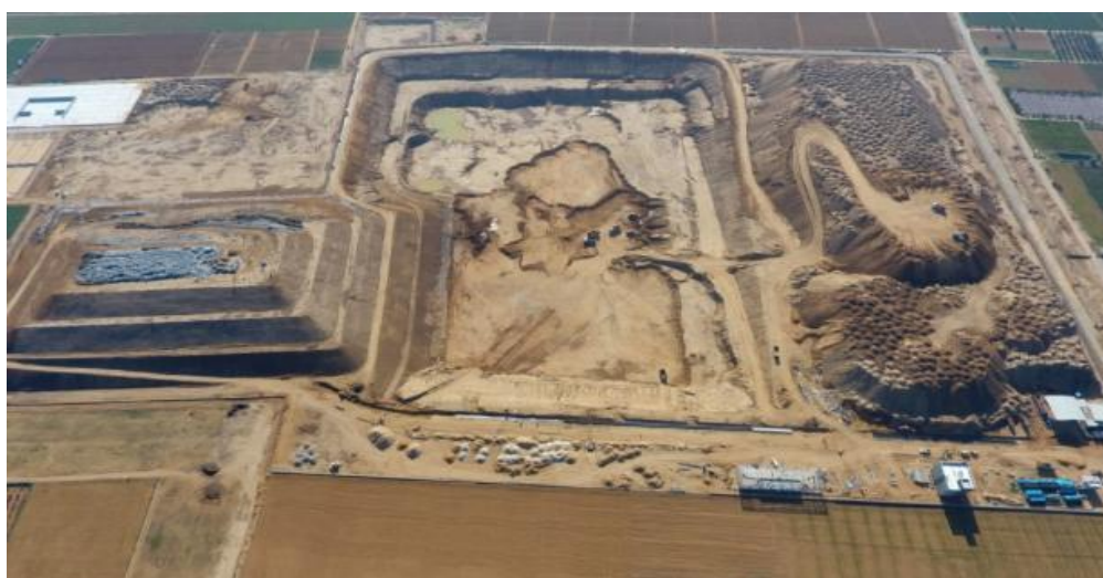
Construction of Al-Fukhari Sanitary Landfill & Rehabilitation of Existing Landfill (December 2018)
