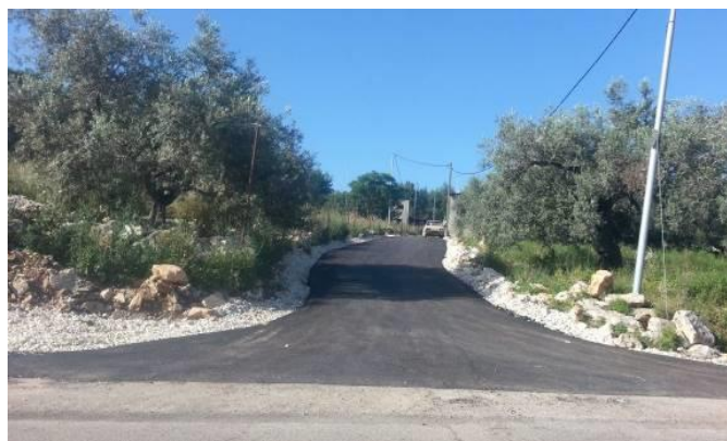
Rehabilitation of Roads / Izbet Al Tabeeb - Qalqilya
