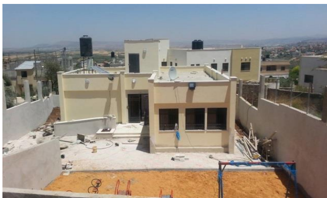
Construction and Finishing of Kinder Garden / Ti'nik–Jenin
