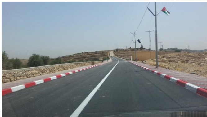
Rehabilitation of Internal Roads/ Um Al Lahim / Jerusalem
