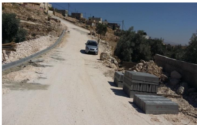
Rehabilitation of internal roads / Twaineh – Hebron
